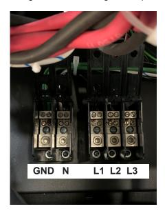
Figure 2.13 – Wiring the AC distribution block
