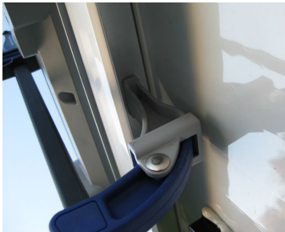
Figure 15. Tip of frame clamp properly seated on inside surface of module frame
