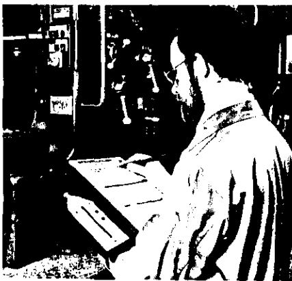
Fig.1. Documentation of measurements taken on site with the Vibration Meter in its folder
