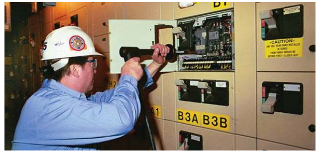
MCCB testing using the HCP2000
