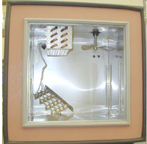
Heater Rack Removal #2
