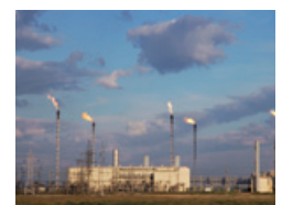
Petrochemical & Chemical industries
