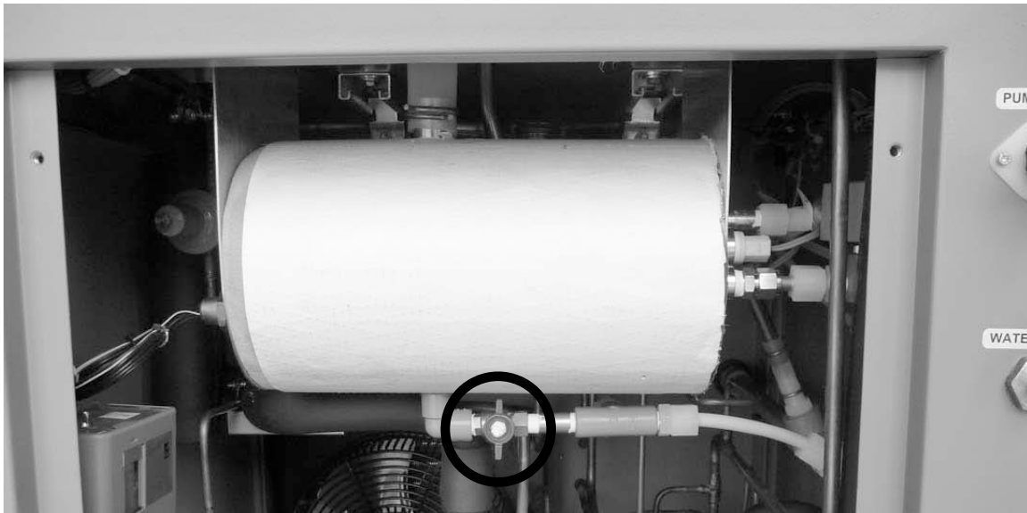
Figure 8-1 – Humidity Drain Valve (shown in the closed, or normal operating position)
