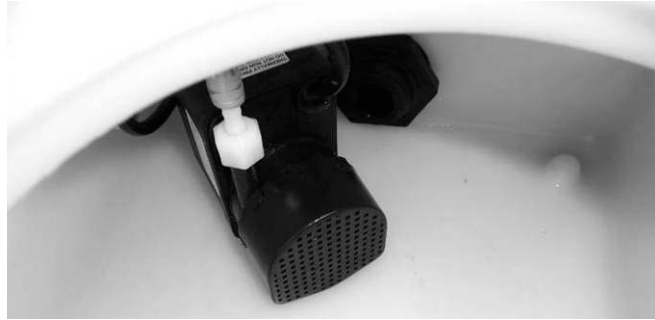
Pump placement in water tank.
