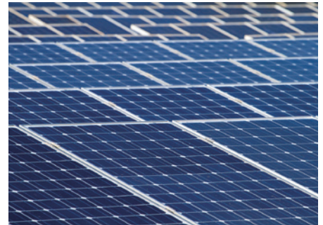
Solar Array Load Testing
