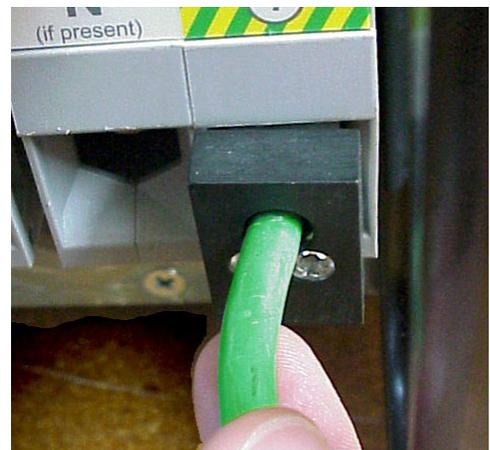
*If your conductors are smaller than 2AWG, use the provided wire size adapters. Insert the stripped wire (top) into the adapter, making sure that the set-screw clamps on the conductor, and that the insulation is fully inside the black insulating block. Then install the adaptor into the gray terminal block. Tug firmly on the wire to verify that it is mechanically secure.*
