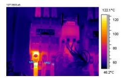
Figure 25.9 An infrared image of indoor electrical equipment (2).
