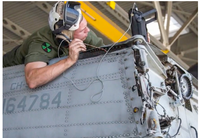
Figure 4: Crack detection around fasteners with MIZ-21C.
