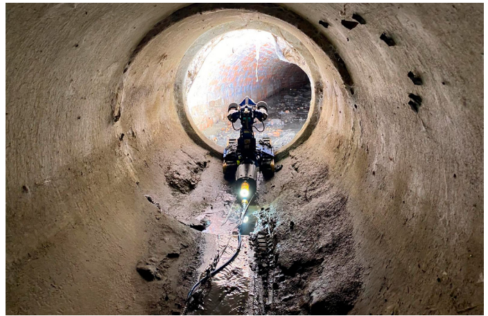
Figure 2: Remote internal pipeline inspection
